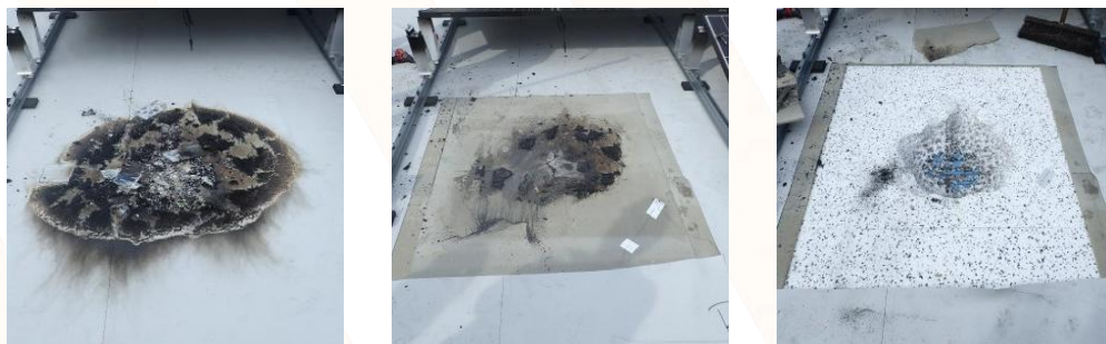
Fig. 5: Fire damage on the roof built-up with an 8 mm Cement board (A2) mitigation layer.
