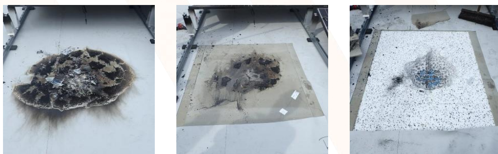
Fig. 6: Fire damage on the roof built up with a 6 mm cement board mitigation layer.
