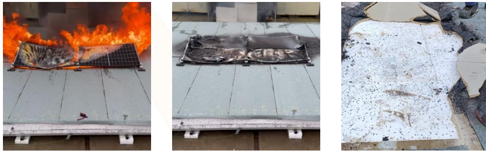
Fig. 7: Fire damage on the roof built-up with bitumen membrane.
