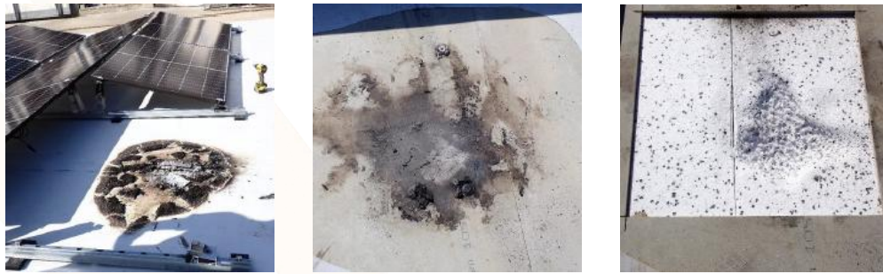
Fig. 4: Fire damage on a roof built-up with a 12 mm Cement board (A2) mitigation layer.
